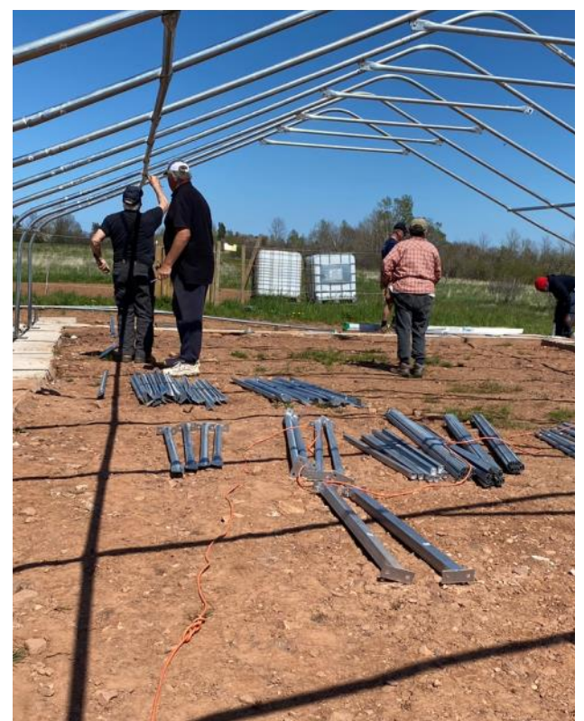
Erecting the greenhouse
