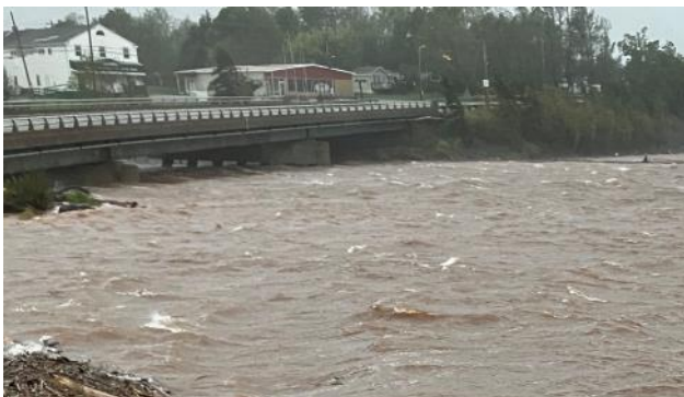
The water nearly up to the bottom of the bridge
