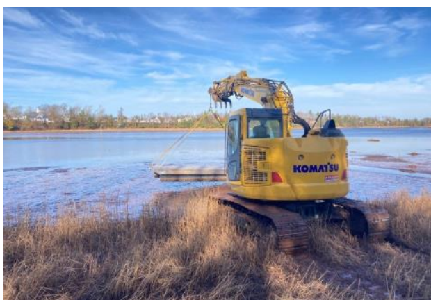
The excavator lifting the docks back into the water
