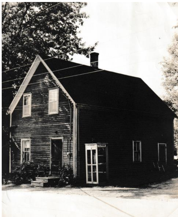
The Munro House with telephone booth
